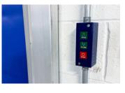
Powered doors include smart motor controller and NEMA1(3) button control.
