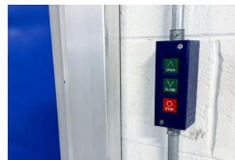
**Powered doors include smart motor controller and NEMA1(3) button control.**
