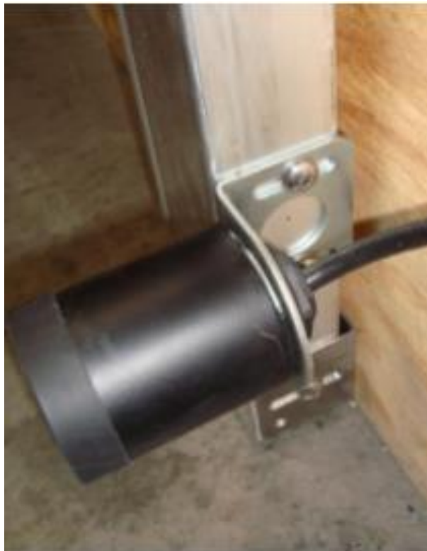
Figure 5: G2 Style Emitter Unit Mounting
