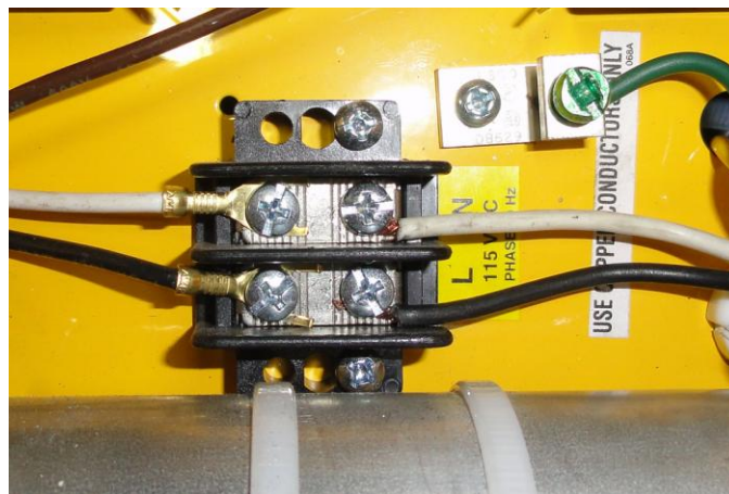
Photo #24 (Power Connections)
