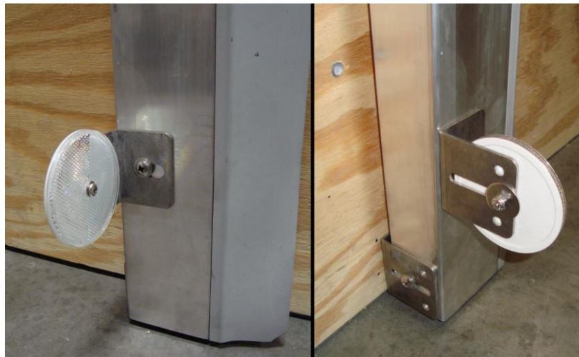
Photo #8 (Reflector Mounting)
