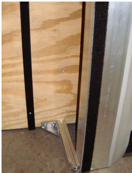
Photo #21 (Velstick Installation)
