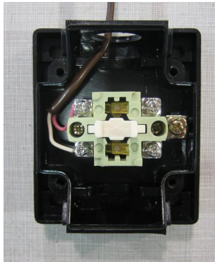
Photo #45 (Single Button Station Wiring)
