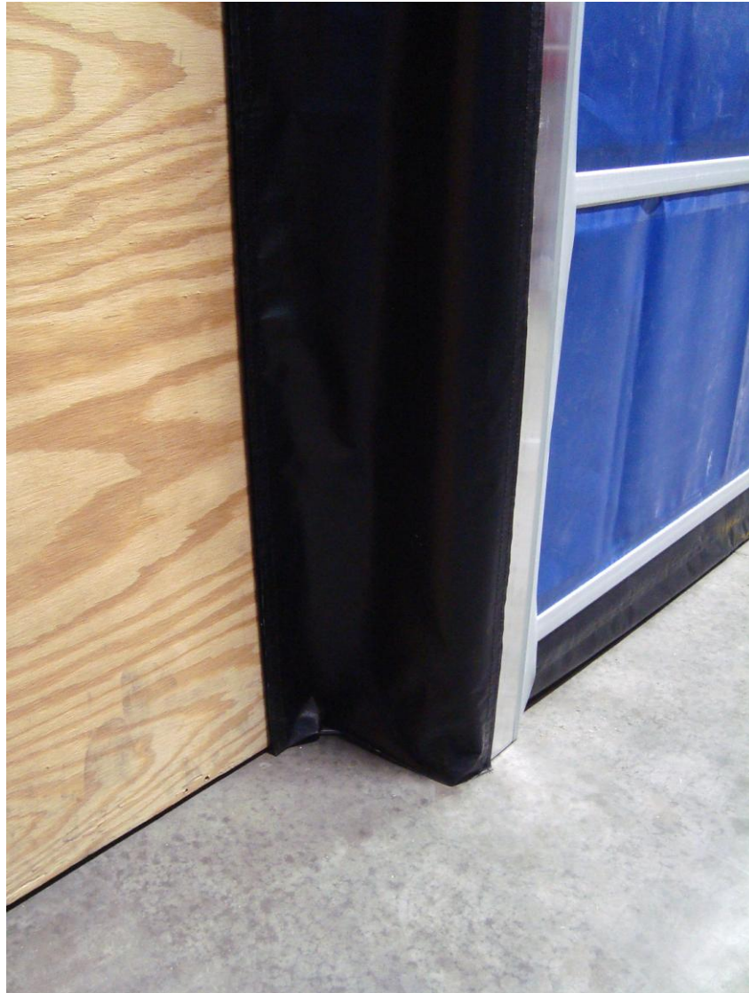
Photo #22 (Side-seal Installation)
