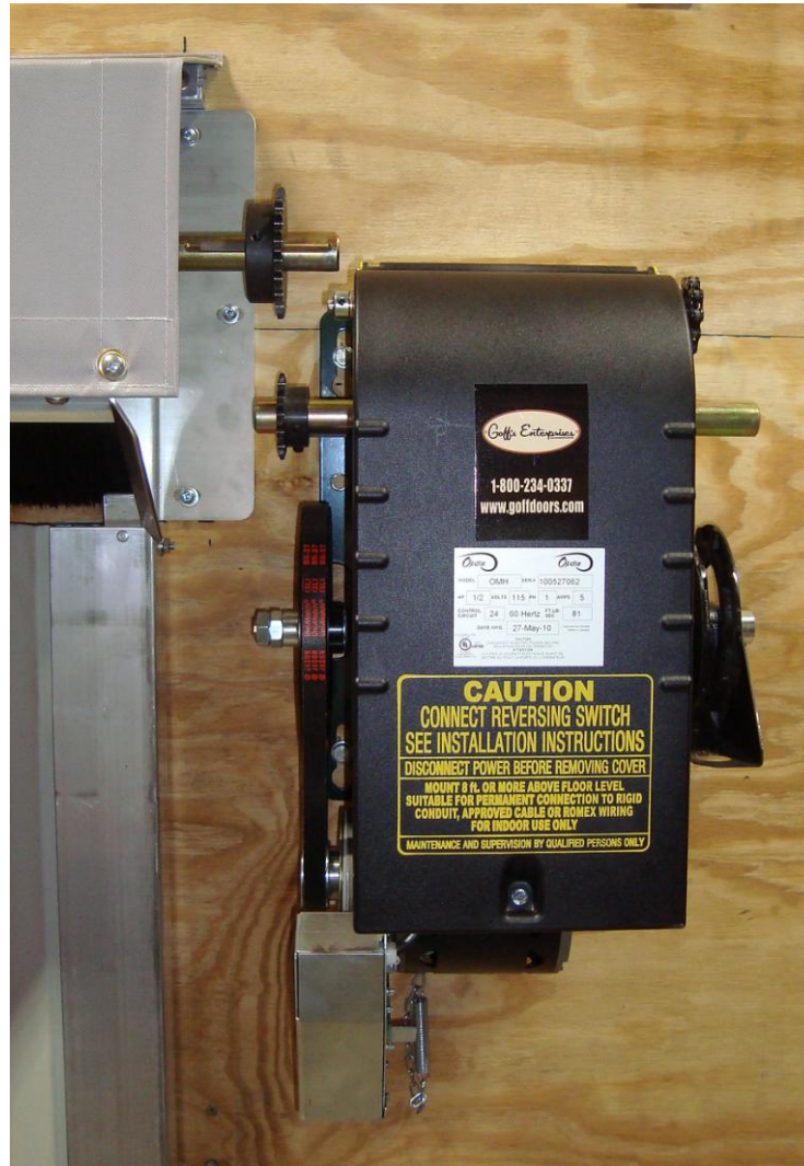
Photo #12 (External Operator Mounting)
