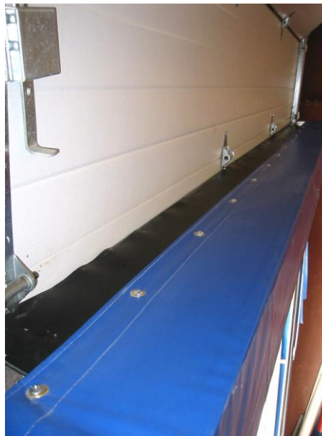
Photo #10 (Flap Seal Deflection)
