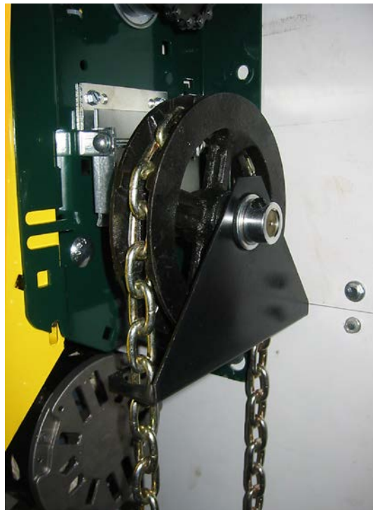
Photo #14 (Hoist Chain Routing)
