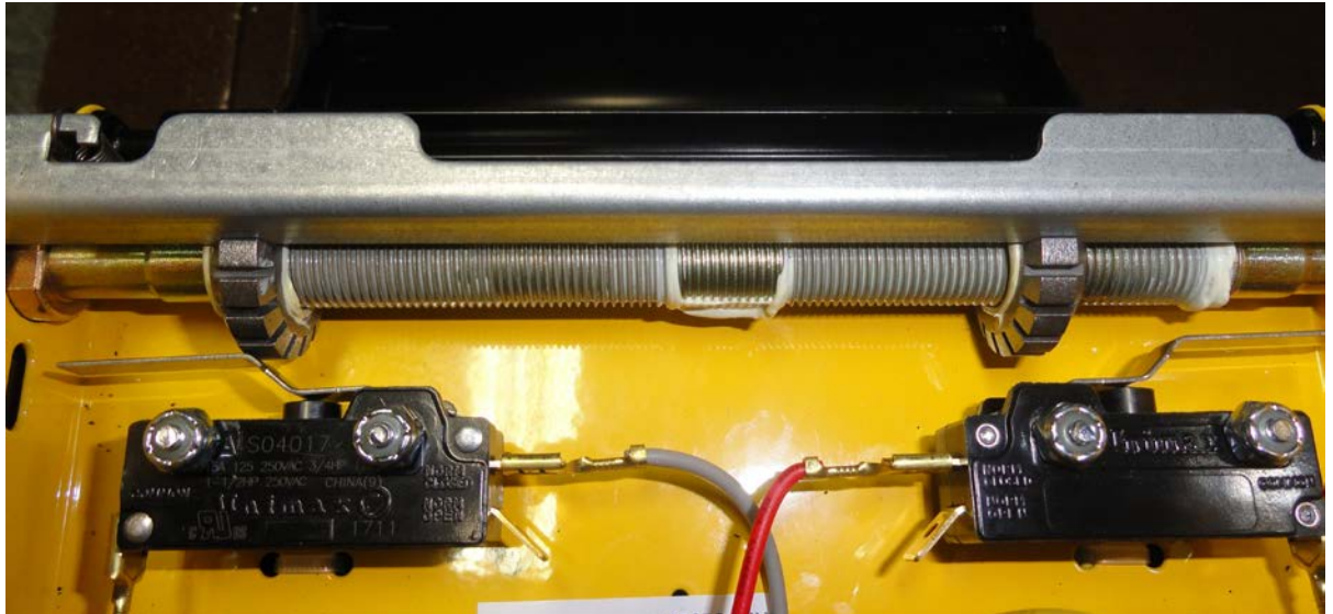
Photo #17 (End Stop Pre-Sets)
