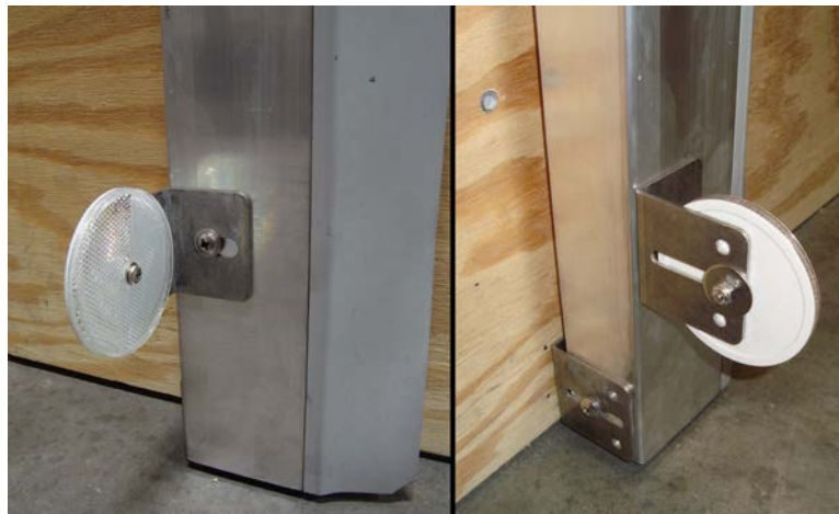
Photo #6 (Reflector Mounting)
