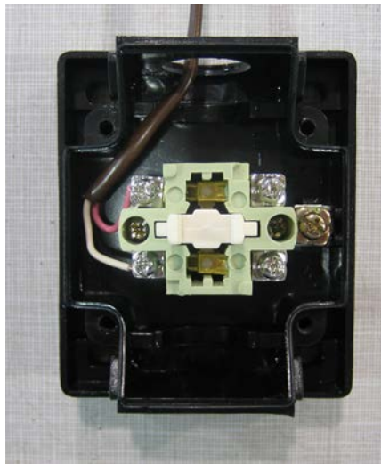
Photo #35 (Single Button Station Wiring)
