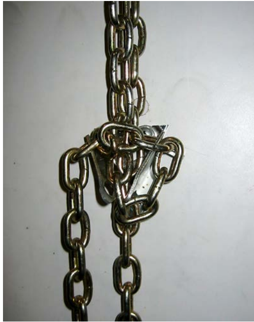
Photo #15 (Hoist Chain Locking)
