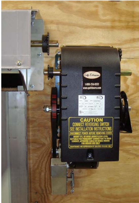
Photo #9 (External Operator Mounting)
