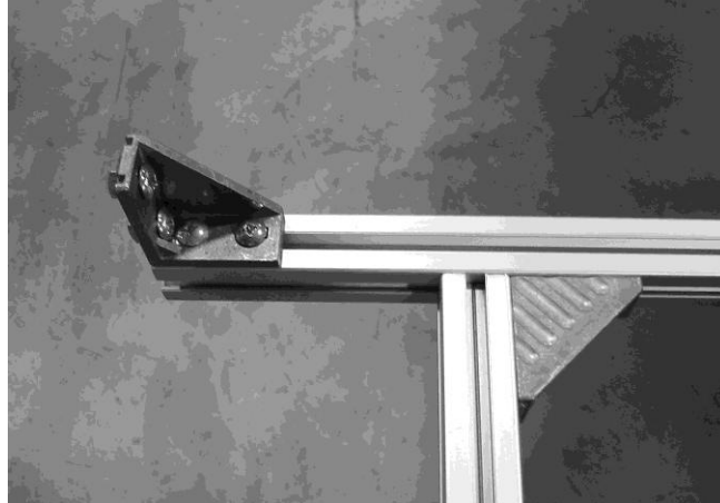
Photo #6 (Leg gusset installation)
