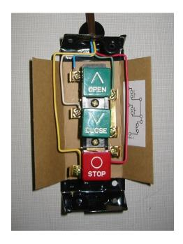
Route the cable through one of the station knockouts and carefully reinstall the cover. Make sure that the cover is installed properly and that the buttons work freely.
