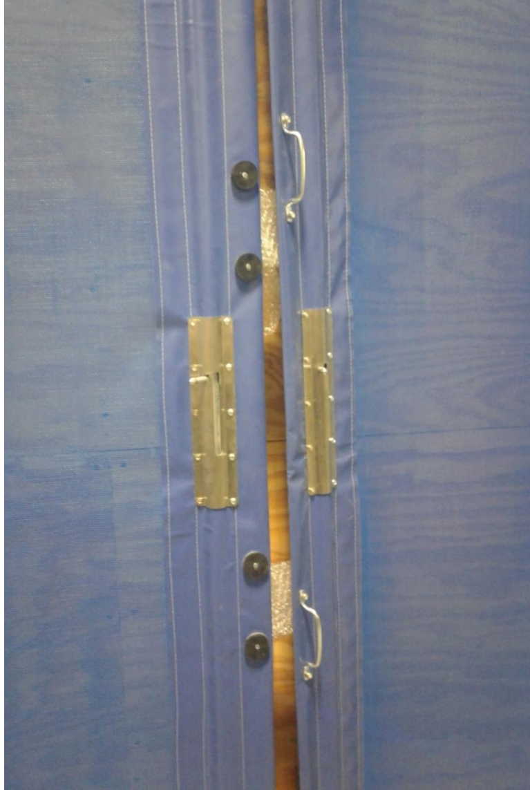
Figure 8 CAM-LOCK ARRANGEMENT (SHOWN NOT FULLY CLOSED)
