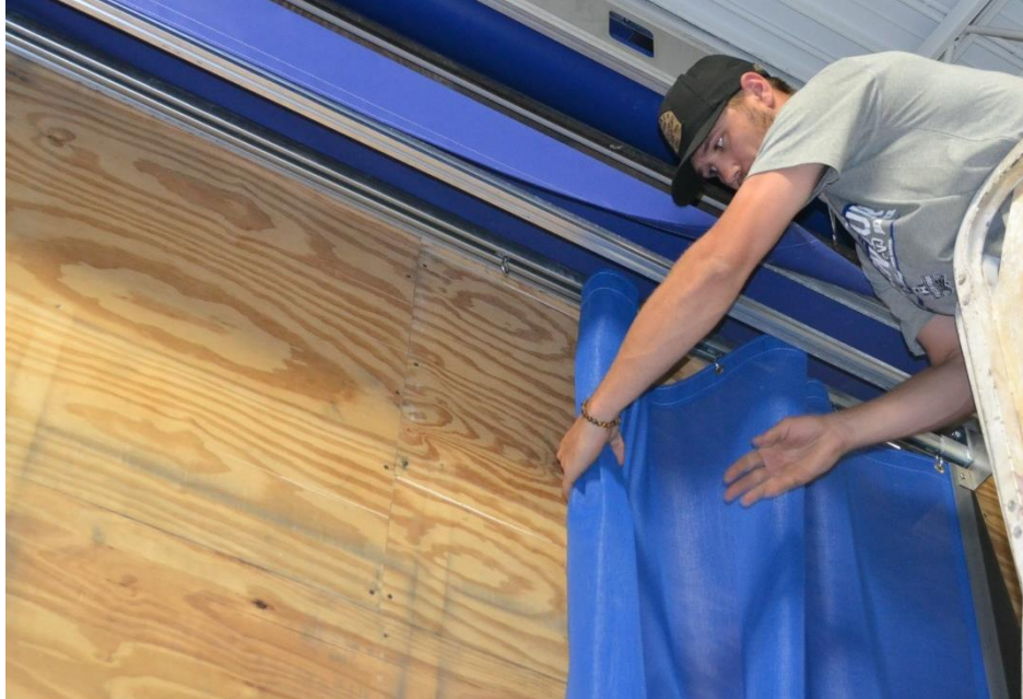
Figure 7 UNROLL CURTAIN, HOOK GROMMETS
