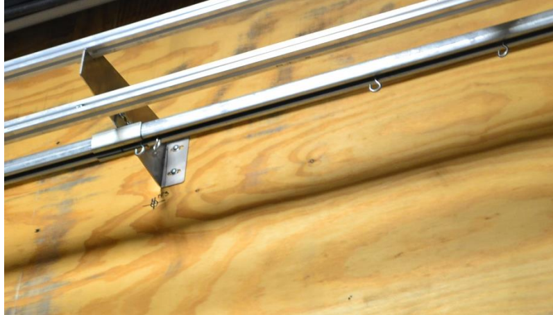
Figure 5 CENTER BRACKET MOUNTING
