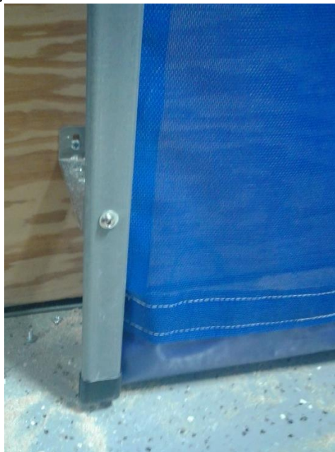
Figure 6 PROJECTION BRACKET ORIENTATION (INSTALLED ON MOUNTING SURFACE)
