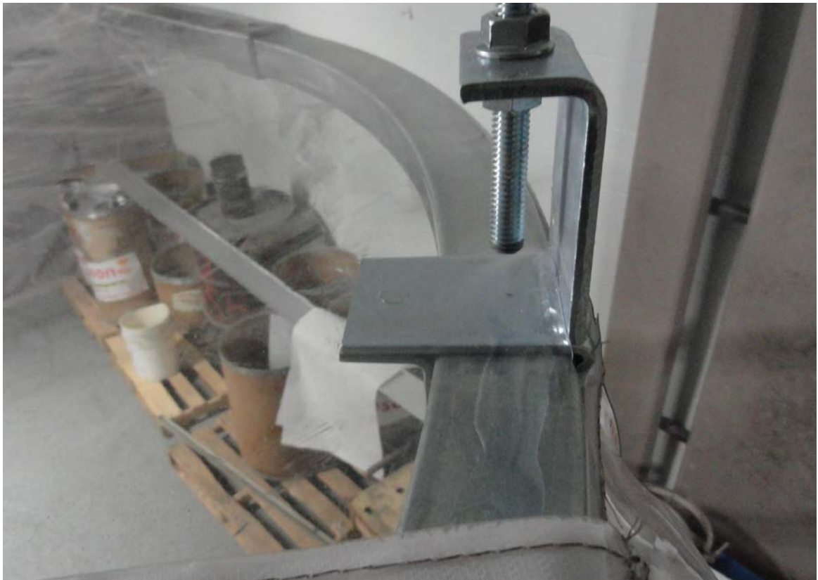
Photo #18 (T-slots installed on Hanger “Ear”)
