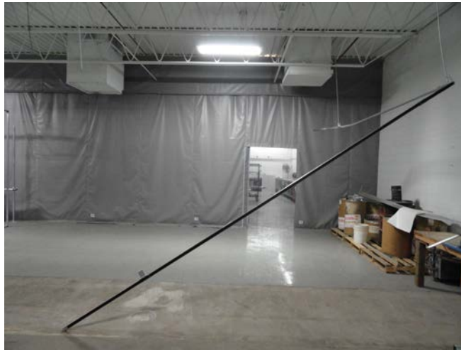
Photo #4 (13' Track Section Installed)
