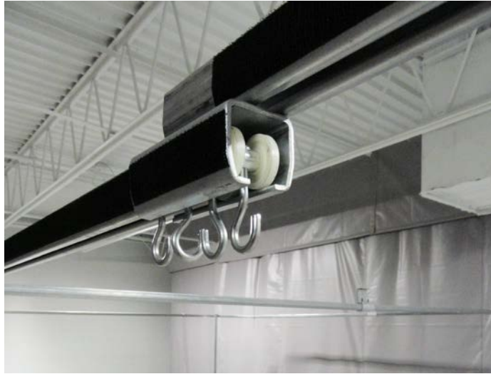
Photo #10 (Roller Installation)
