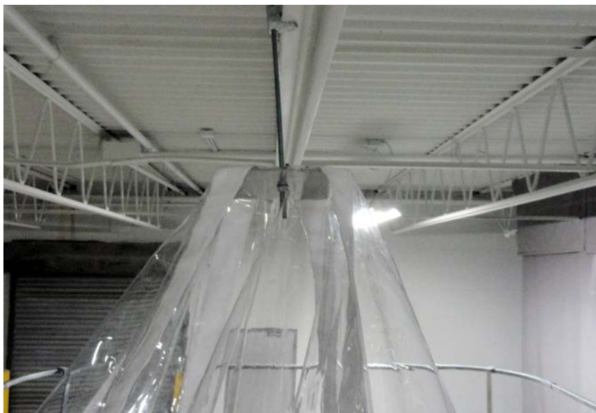
Photo #16 (Hanger Plate Initial Suspension)
