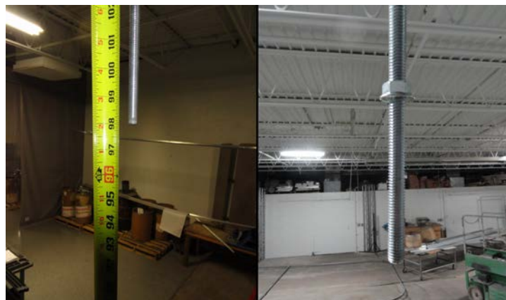
Photo #1 (Threaded Rod Drops)
