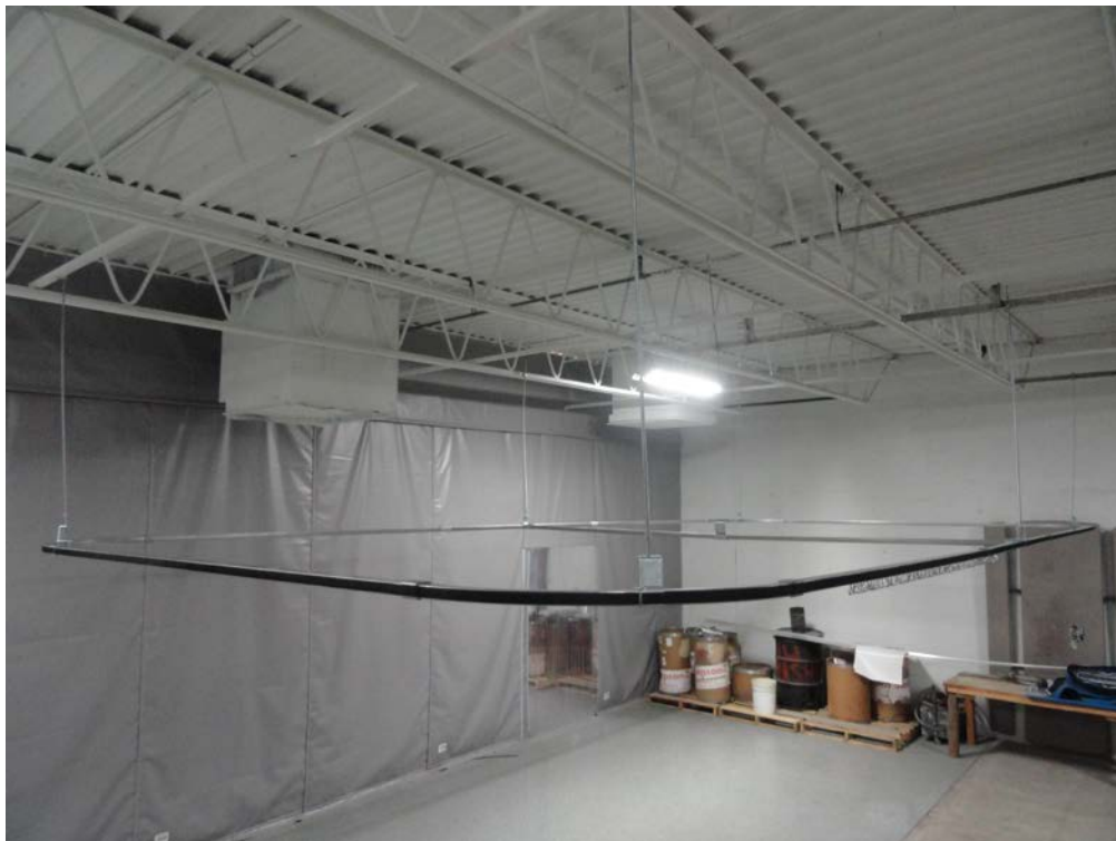
Photo #11 (Completed Track Assembly)
