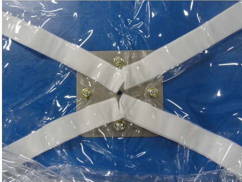
Photo #15 (Hanger Plate Installation)
