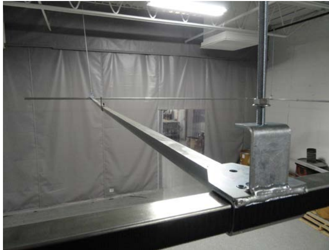
Photo #8 (Center Track and Hangers Assembly)
