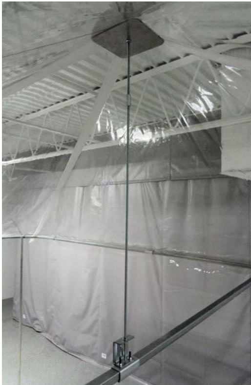
Photo #20 (Center Span Threaded Rod Support)
