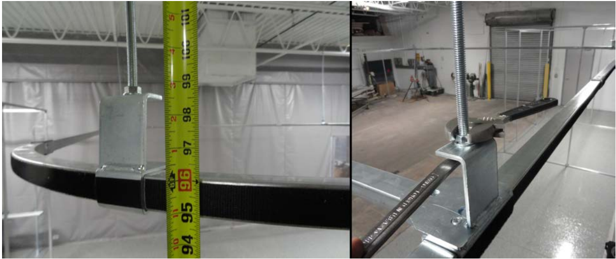
Photo #12 (Setting the Track Height)
